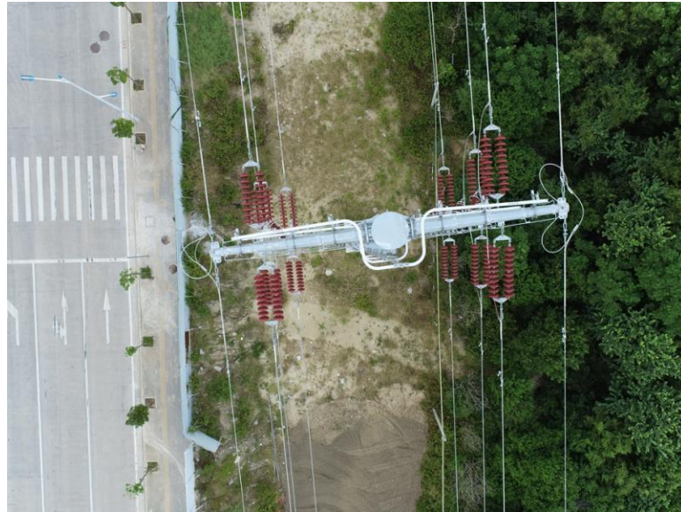
Figure: View from the top of a power pylon to record a waypoint (you can adjust the gimbal to be -90° and adjust the aircraft position)
