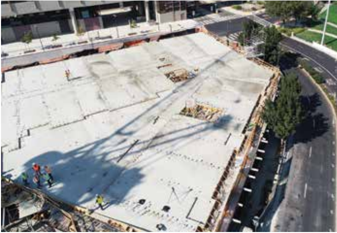
Fig. 2: The podium-level slab included many protruding anchor rods (aerial photo courtesy of BKF Engineers)
