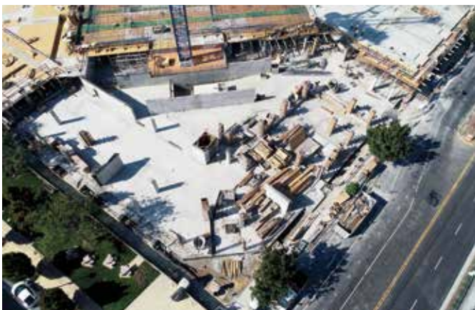
Fig. 3: Ten targets were placed at various locations on vertical surfaces (concrete walls and columns at the ground level) for participants to determine their point coordinates. The reference target point coordinates were obtained using a total station at three locations. Ten targets were also placed at various locations on the horizontal concrete surface at the podium level (aerial photo courtesy of BKF Engineers)
