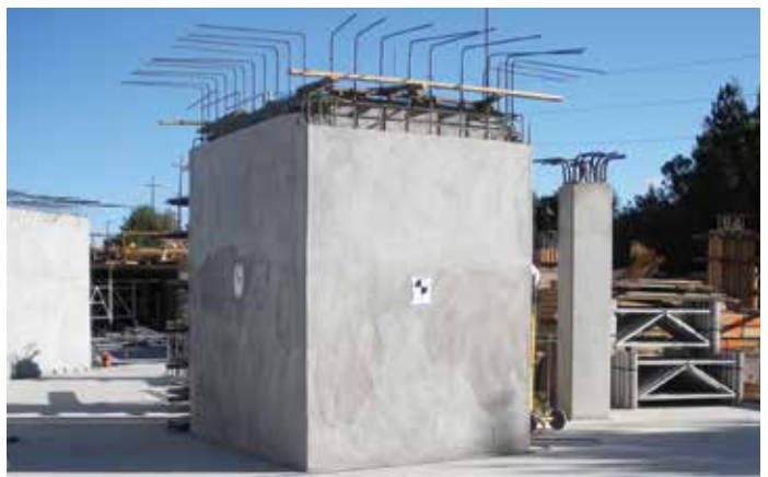
Fig. 3: Ten targets were placed at various locations on vertical surfaces (concrete walls and columns at the ground level) for participants to determine their point coordinates. The reference target point coordinates were obtained using a total station at three locations. Ten targets were also placed at various locations on the horizontal concrete surface at the podium level (aerial photo courtesy of BKF Engineers)
