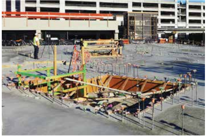
Fig. 2: The podium-level slab included many protruding anchor rods (aerial photo courtesy of BKF Engineers)
